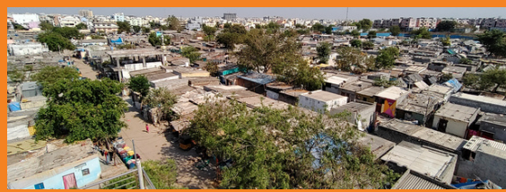
A large portion of the urban population in cities of the global South live under housing conditions that render them additionally vulnerable to the impacts of extreme heat (Image Credit: Goutham Raj Konda).
